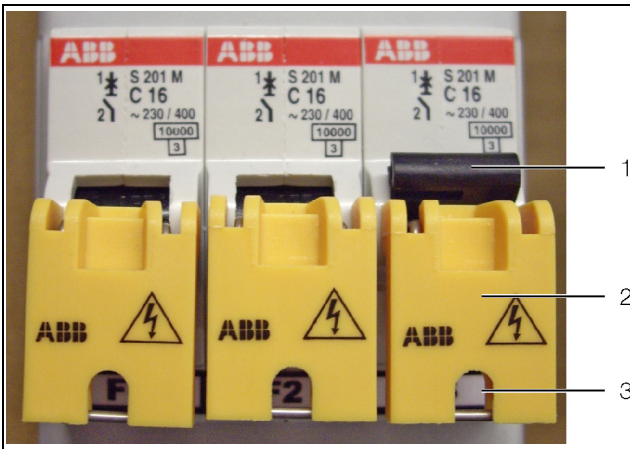
Fig. 10: Securing the lockout
